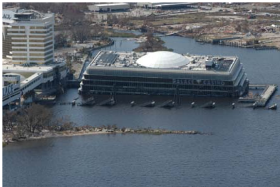
The Palace Casino After Damaged by Hurricane Katrina
